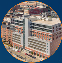
22 BOSTON WHARF ROAD Boston, MA 123,875 SF
