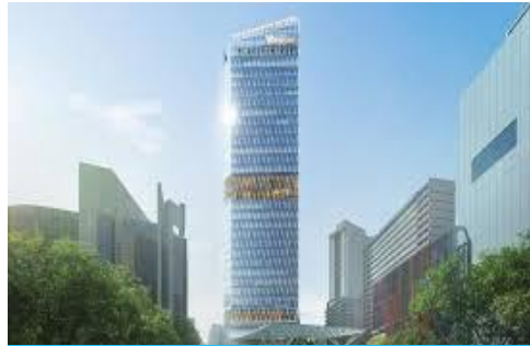
Keppel South Central 10 Hoe Chiang Road
